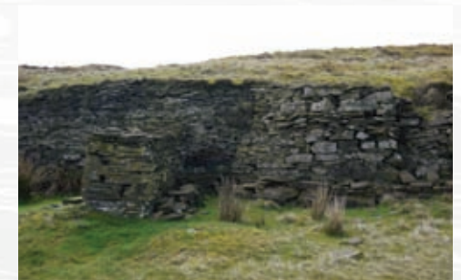
Judd Walls on Oxenhope Moor. These walls made from discarded stone from the quarry and are built to retain waste material from the quarrying activity
